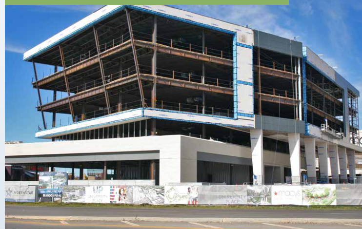
5 STORY BUILDING UNDER CONSTRUCTION 2016 OCCUPANCY
