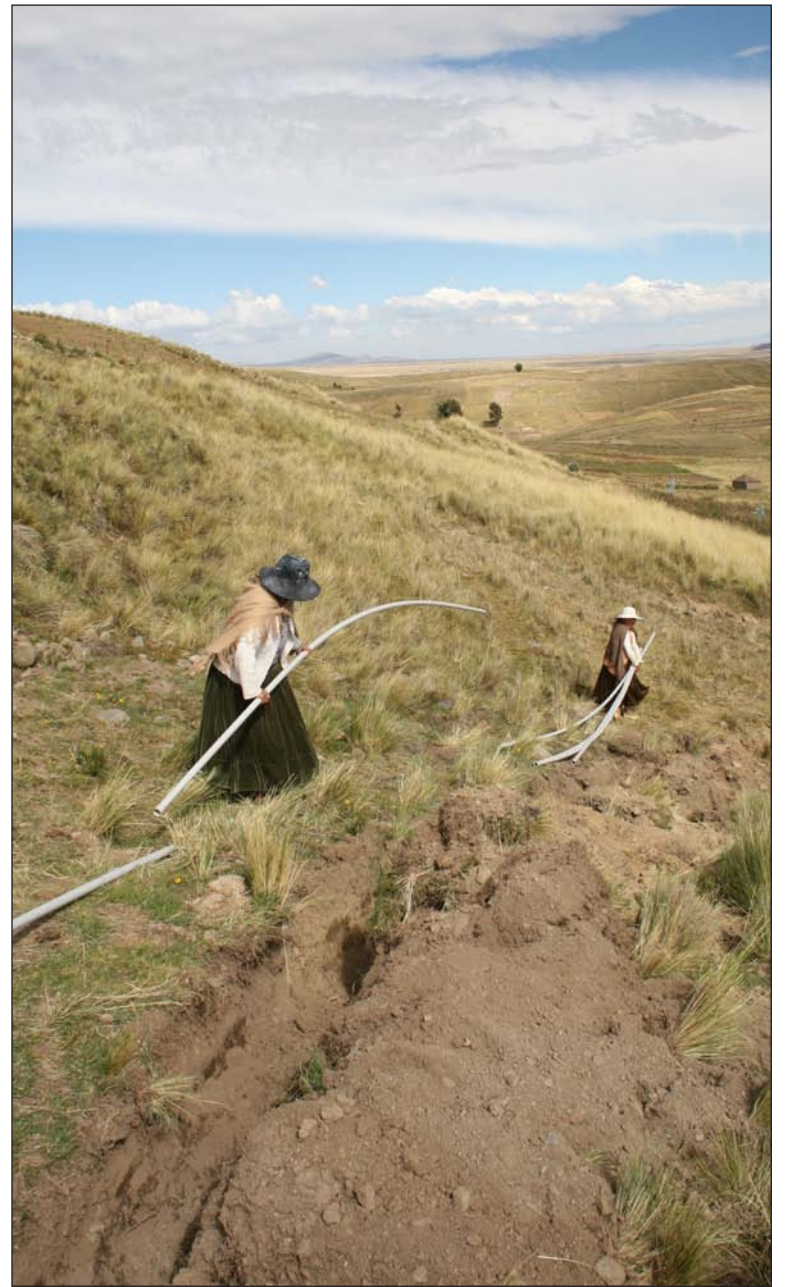
Bolivian villagers join with Salt Lake's Wheeler Machinery volunteers to lay pipe and bring fresh water to their homes for the first time.
