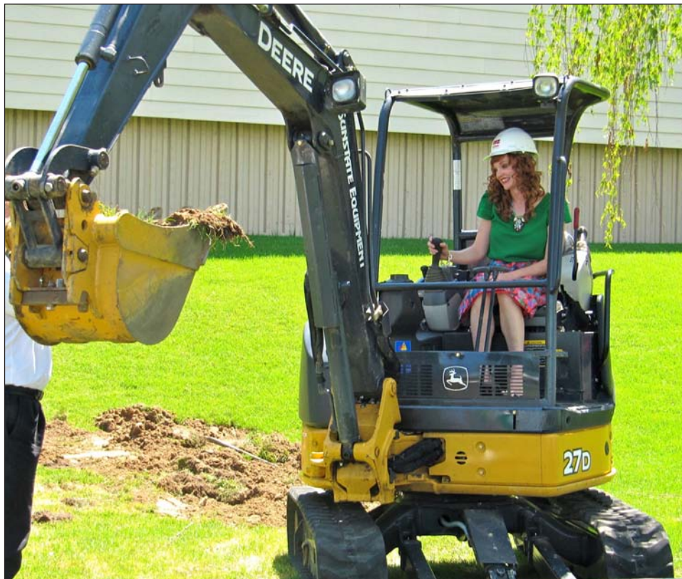
Dr. Megan Grunander, an Ogden Clinic general surgeon, takes the first socop as doctors break ground for a new $9 million, 41,000 square foot medical campus on Harrison Blvd.
