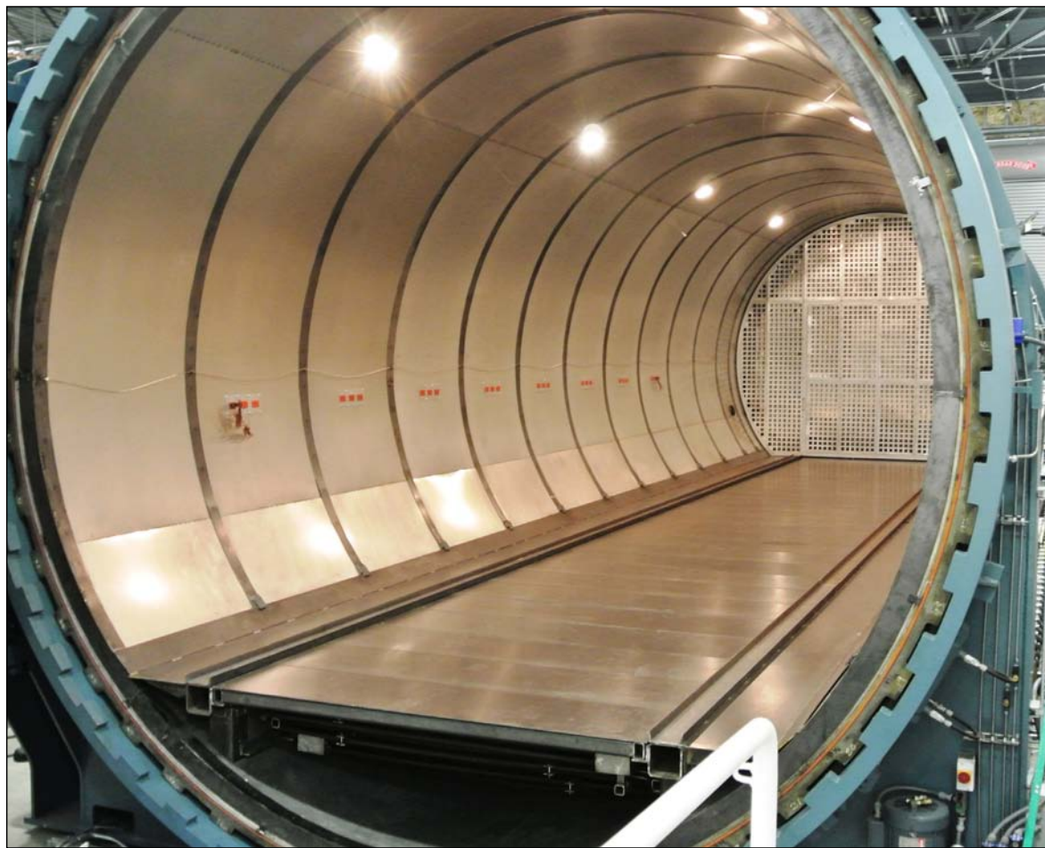
An autoclave stands at the ready at Exelis Aerostructures' new composite design and manufacturing facility near the Salt Lake City International Airport. The device is one of several in the now-operational 250,000-square-foot facility, which focuses on producing composite structures used in military and commercial aircraft.
