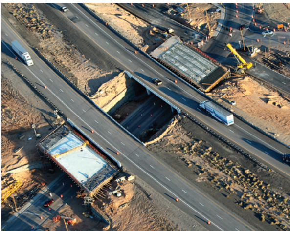
Mesquite Nevada: First ever accelerated bridge construction in the state saving $10 million in costs.
