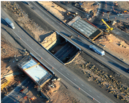
Mesquite Nevada: First ever accelerated bridge construction in the state saving $10 million in costs.
