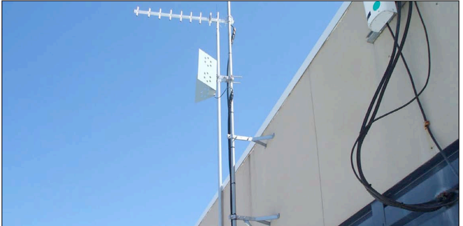
Distributed antenna systems begin with a head-end antenna that receives the radio frequency (RF) signal from the wireless carriers and distributes them through buildings that would otherwise have poor cellular reception.
