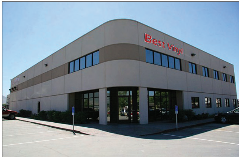
Best Vinyl's new Utah County facility will be twice as large as its former location in American Fork.
