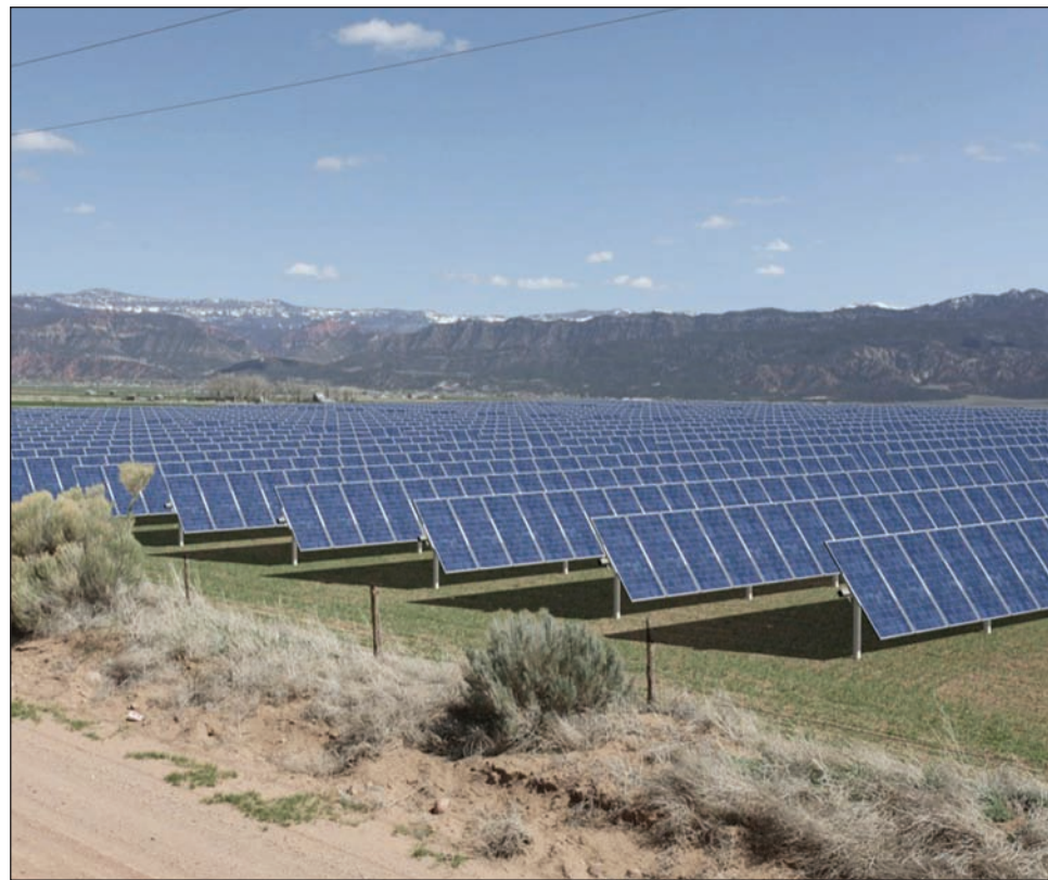
About 350,000 of these photovoltaic panels — shown in this artist's composite picture of the actual site — will soon cover 650 acres in Parowan in Iron County. The installation will be the largest solar farm in Utah and among the top 12 in the United States.
