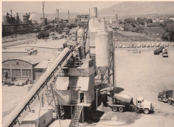
First Geneva Rock Products Batch Plant
