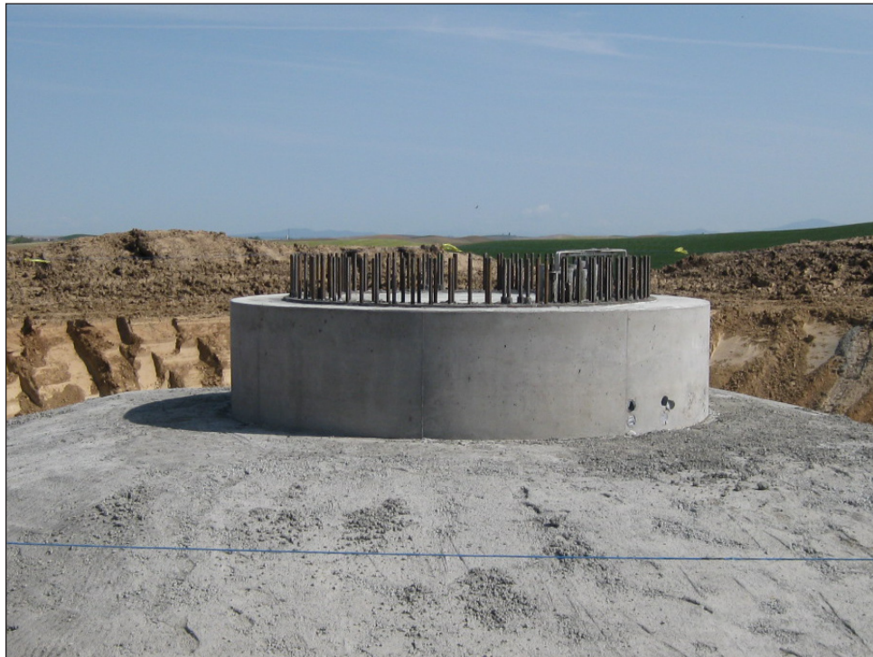
Footings are being poured for the massive wind-powered turbines being installed at the Blue Mountain Utah wind energy site near Monticello. RMT Inc., a Wisconsin-based construction company, began work on the Greenbriar Capital Corp. project earlier this month.
