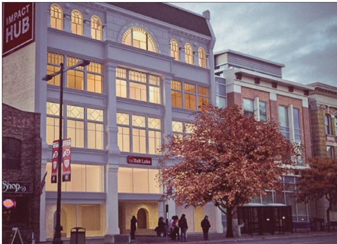
Impact Hub Utah's permanent home is undergoing remodeling in downtown Salt Lake City.
