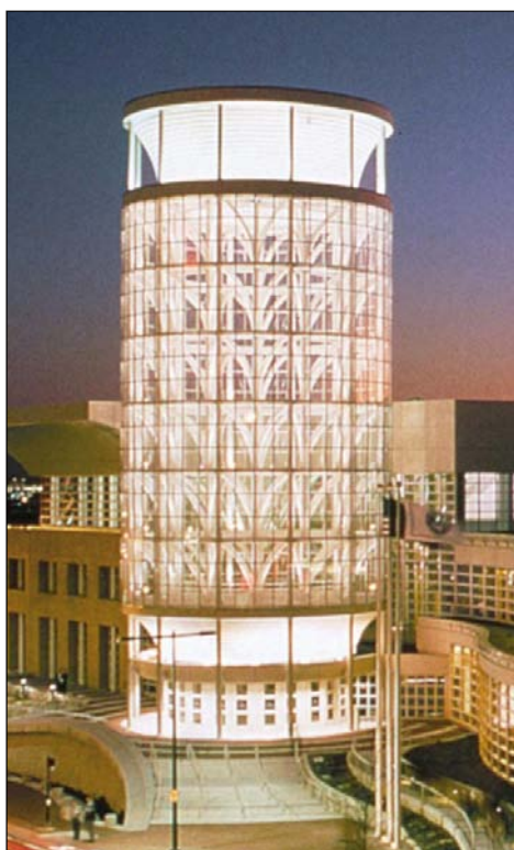
The legislation that paved the way for a new convention center hotel in Salt Lake City calls for the facility to be built in close proximity to the Calvin L. Rampton Salt Palace Convention Center.
