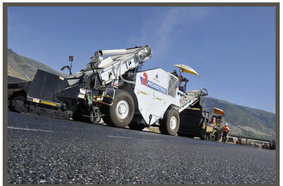
Staker Parson’s work on I-15 from Farmington to Gordon Avenue was awarded as the best asphalt pavement project in the US in 2011.
