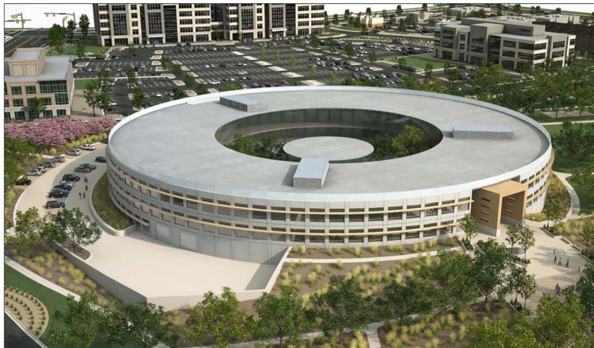
Overstock.com has released plans to build a 230,793-square-foot office complex near Bingham Junction in Midvale. A groundbreaking was held last week and opening is set for summer 2016.
