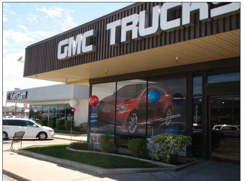
Garff's GMC/Buick dealership in Ogden is located in a 20-year-old building that is in need of major improvements.
