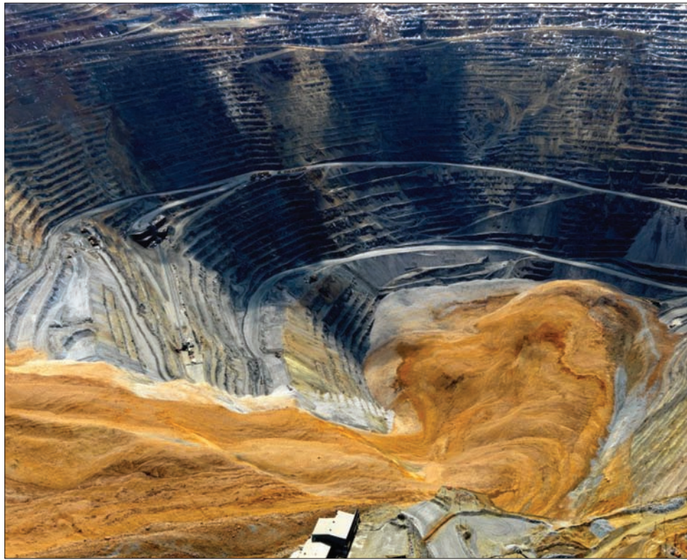
The massive landslide in the Bingham Canyon Mine of Kennecott Utah Copper is shown shortly after it occurred in April. The company has now cleared enough of the debris and rebuilt infrastructure in order to resume full production.
