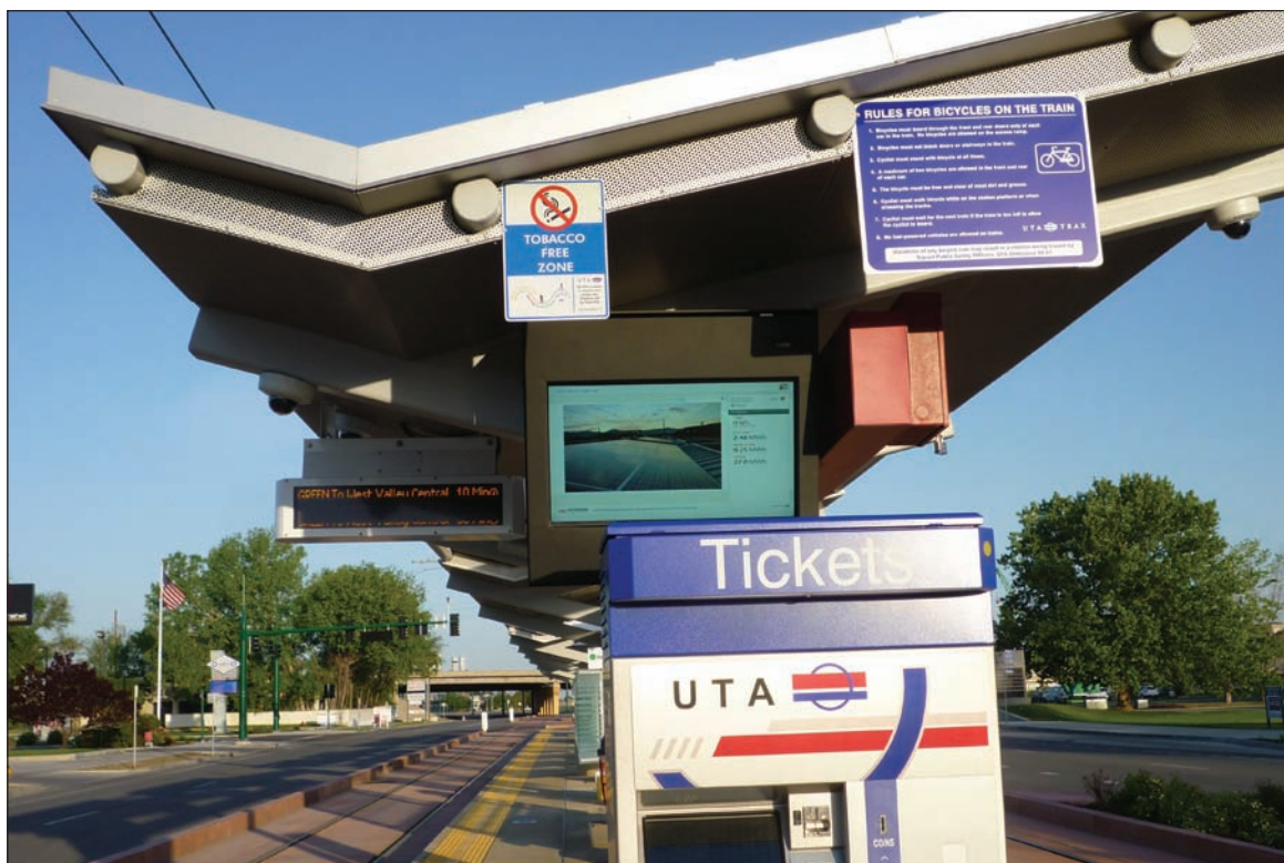
The new TRAX airport line station on North Temple nearest the airport along with three other stations, are fully self-powered through solar microinverters installed on the roofs of the stations.
