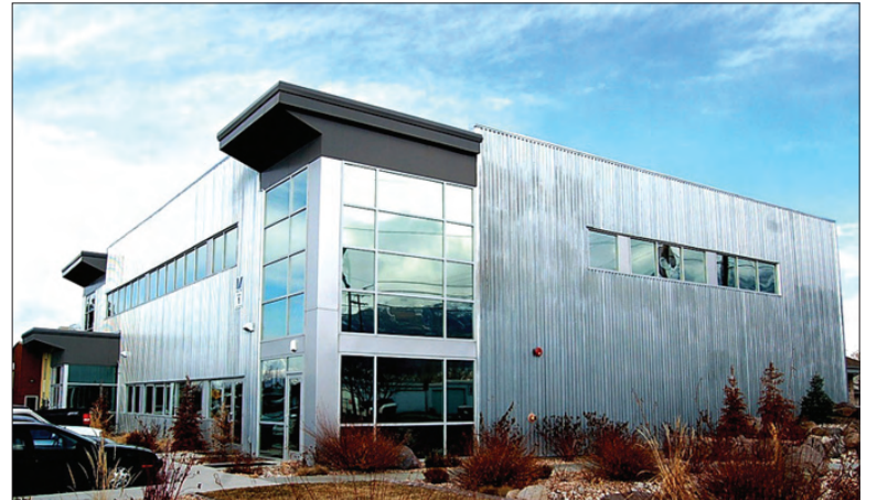
Moxtek plans to construct an 83,000 square foot building at its current five-building Orem campus.
