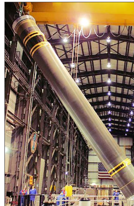
A composite casing is hoisted into place at Northrop Grumman's Bacchus Utah plant. The company has received an incentive from the Utah Inland Port Authority to build a composite materials manufacturing plant at the inland port's Northwest Quadrant area in Salt Lake City — the first such incentive awarded by the UIPA.
