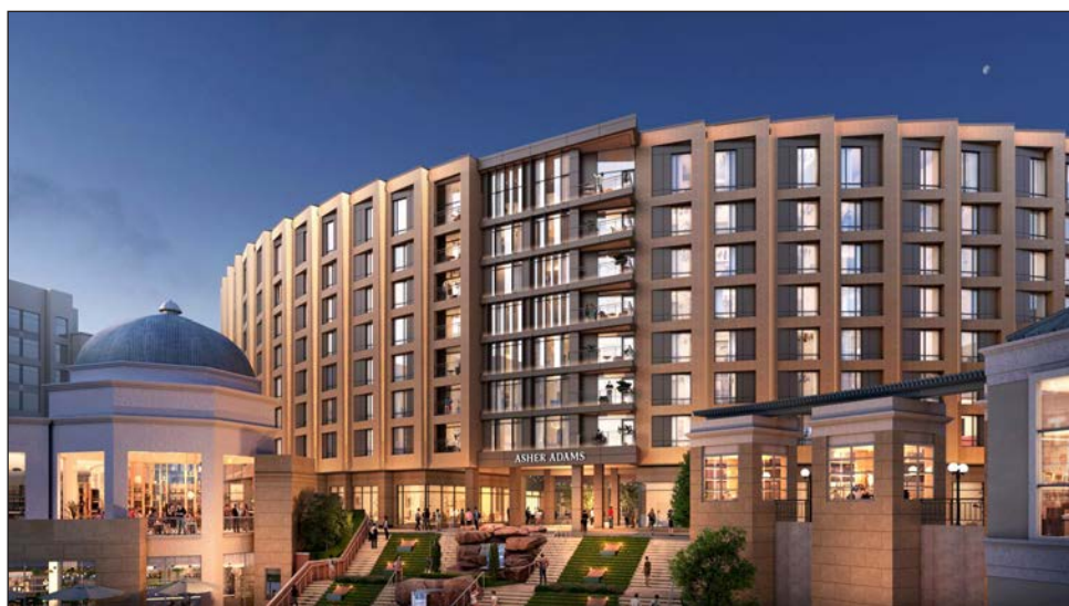
A view of the new Asher Adams hotel at The Gateway in downtown Salt Lake City shows the new construction part of the facility. The opposite side of the 225-room hotel will be a rebuild of the historic Union Pacific railroad station facing 400 West.
