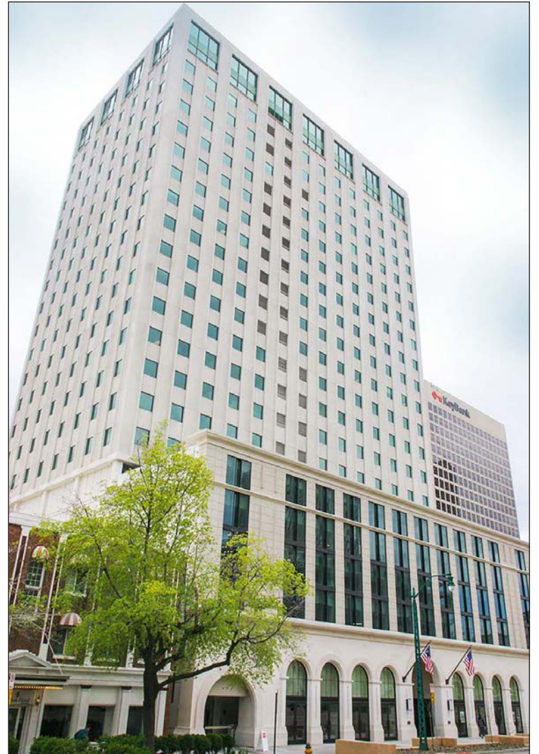
Downtown Salt Lake City's South Temple Tower has been purchased by real estate giant Hines. The company plans to convert the current office structure into a 255-unit luxury residential building.
