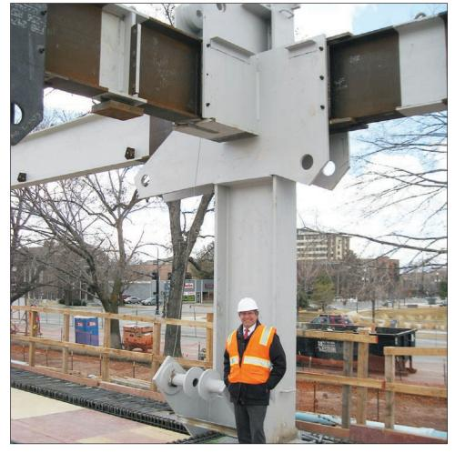
The steel "skeleton" of Salt Lake City's Public Service Building, shown here during construction, is designed to support the structure and insure "immediate operation" in the event of a earthquake. The design worked and there was no downtime during March's 5.7 magnitude shaker.
