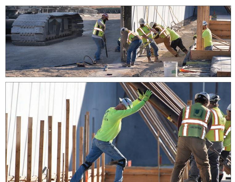
Workers from Jacobsen Construction work to position concrete tilt-up panels as they complete the warehouse portion of doTerra's new distribution center.
