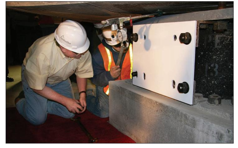
Construction workers examine a base isolator that was installed as part of a major seismic renovation to the Utah State Capitol.
