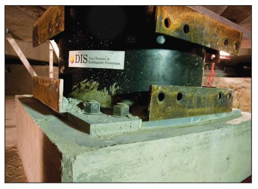
Pictured is one of the base isolators that was installed as part of a major seismic renovation to the Utah State Capitol.
