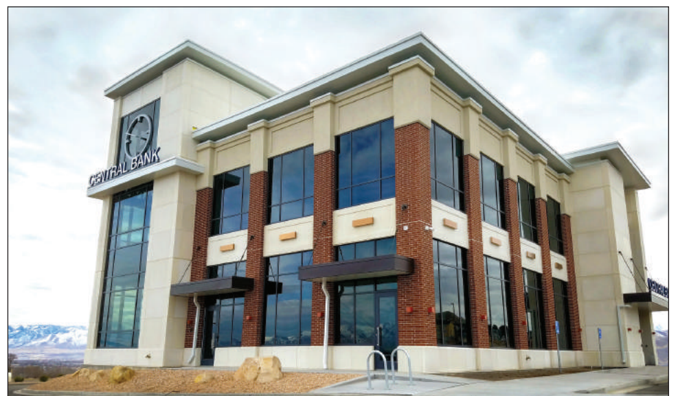
Central Bank branch at Traverse Mountain in Lehi.
