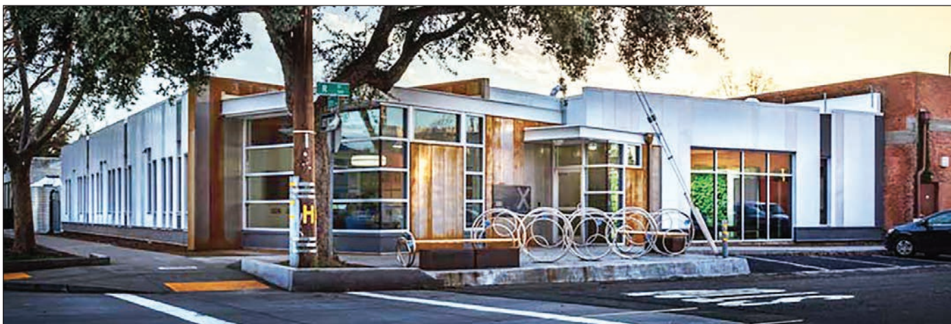
The Sacramento offices of Salt Lake City's Architectural Nexus could be the world's first rebuild project to meet the Living Building Challenge.
