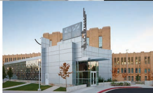
Historical restoration of Ogden High School in Ogden Utah is completed
