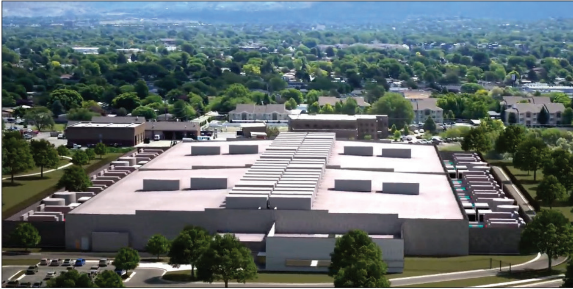
Cirrus Data Services is developing the first phase of its View 78 Data Center campus in Midvale. The data colocation facility will include a 32-megawatt wholesale and hyperscale center in the 224,000-square-foot building
