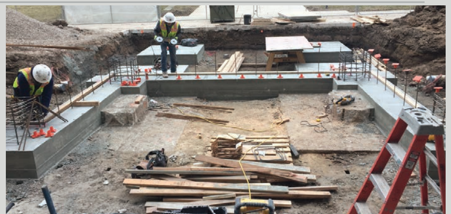
During demolition of the existing building, Big-D recycled more than 95% of the materials.
