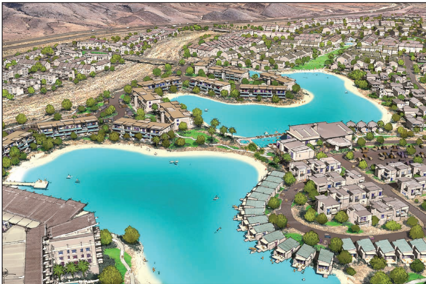
A massive master-planned community in the southern part of St. George in under construction near the Arizona state line. Recreational facilities will be a large part of the development that will also include a resort hotel, retail areas and as many as 10,000 residences.
