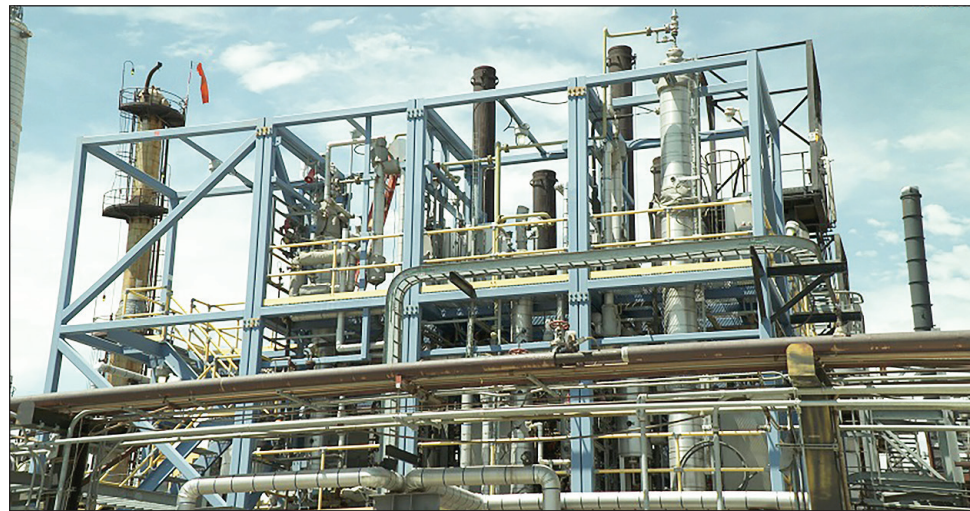
The alkylation unit at the Chevron Salt Lake City oil refinery will be part of the equipment revamped as the company converts the facility to produce low-sulfur Tier 3 fuels. Chevron expects the reconfiguration to be complete by the end of 2019. Photo courtesy of Honeywell UOP
