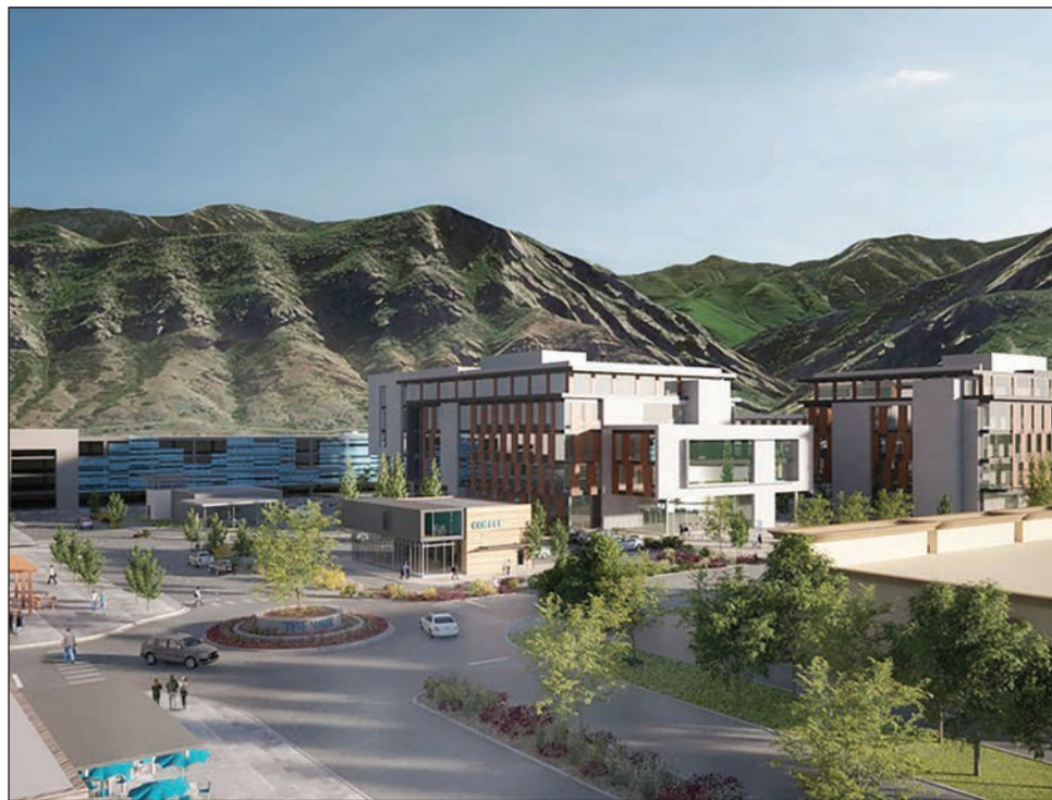
Work is underway on a 1.1 million-square-foot, $161 million project called The Mix at River's Edge on University Parkway in Provo. The development, which replaces the Plumtree Plaza , will contain retail, office space, family dwellings and a high-rise hotel.
