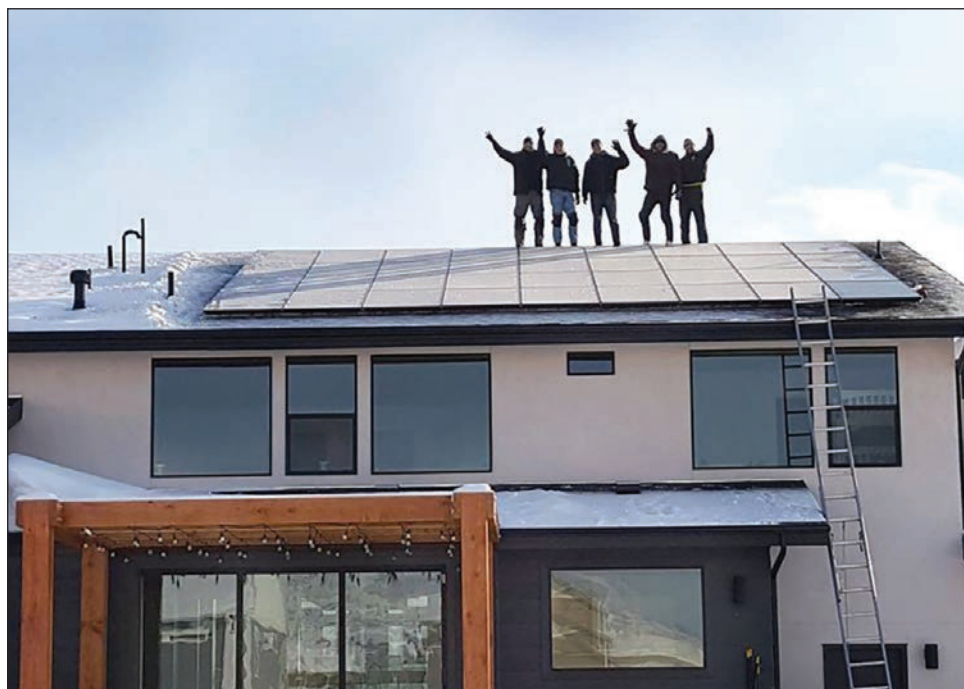
Workers take a break during a recent rooftop solar installation in Highland. Utah ranks seventh in the nation per capita for people employed in the solar industry, according to a report from the Solar Foundation.
