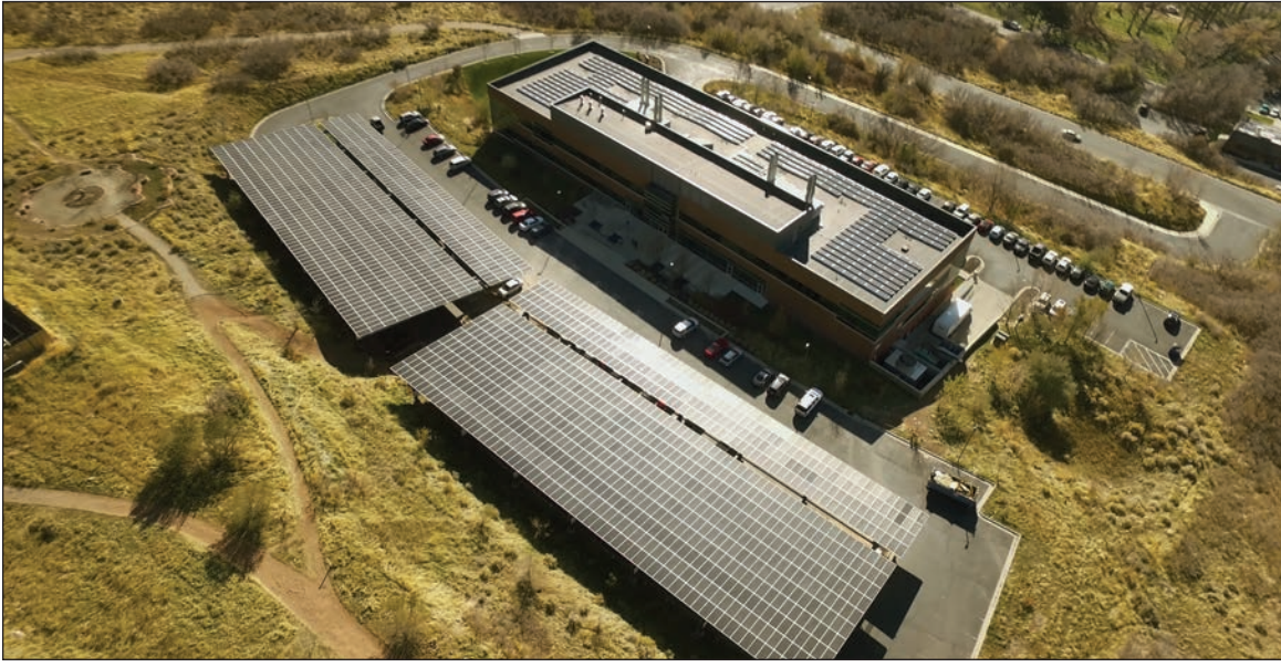
A new solar array on the rooftop and parking canopy of a University of Utah Research Park building at 383 Colorow Way came on line last month and will offset about 27 percent of the facility's energy consumption.
