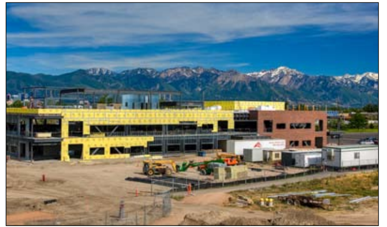
Drawbridge Realty Trust has begun construction on a 88,461 square foot research and office building at the previously undeveloped Airport Technical Park on Salt Lake City's west side.
