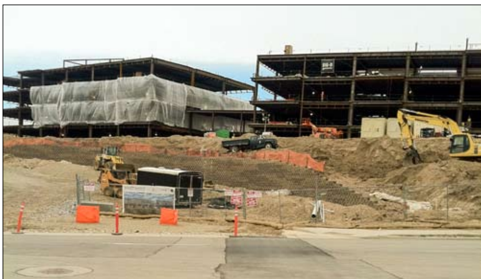
Construction continues on an expansion project undertaken by software company Xactware Solutions Inc. The expansion includes a 210,000 square foot building at Traverse Mountain in Lehi that will serve as the company's headquarters. The company last year was awarded a tax credit from the Governor's Office of Economic Development board of nearly $32.3 million over 20 years, tied to the creation of 859 high-paying jobs.
