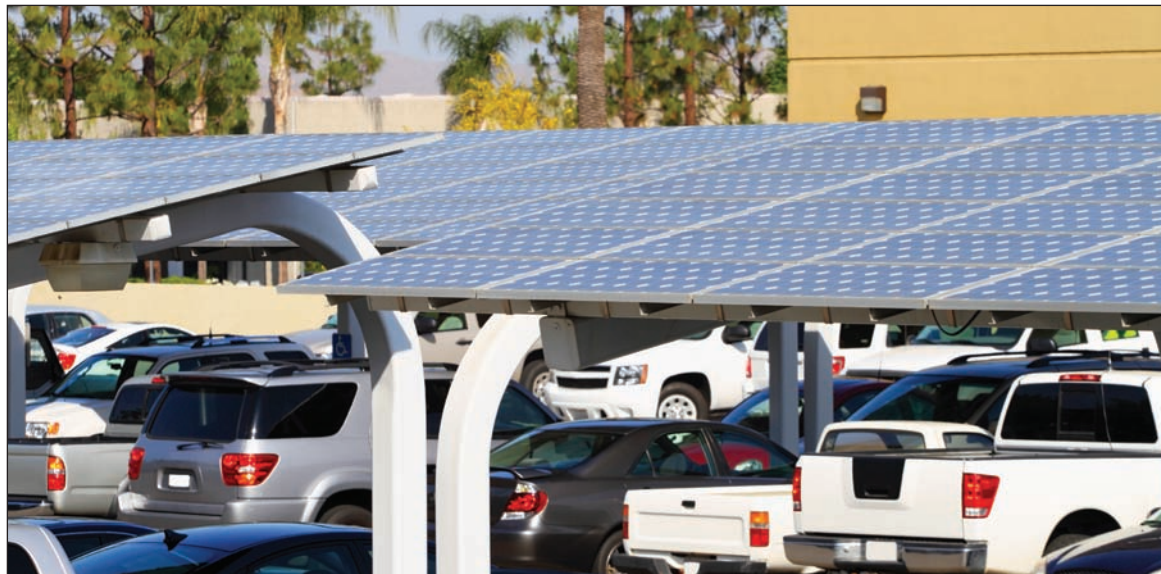
A solar canopy at the Hunt Electric offices in Salt Lake City is the first project financed under the PACE program in Utah.
