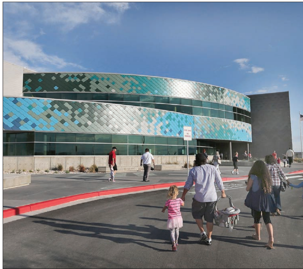
Investment in state-funded projects such as the Odyssey Elementary School in Woods Cross is one of the reasons local engineering firms are doing well. Consulting engineers Van Boerum & Frank Associates delivered a net-zero design for the modernistic building.
