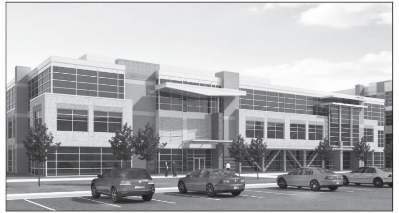
Ground has been broken for the building at Hill Air Force Base's Falcon Hill National Aerospace Research Park where Lockheed Martin will compete for the contract to develop the nation's new intercontinental ballistic missile system.
