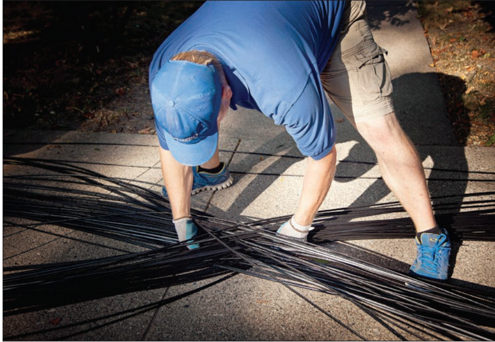
A worker lays out fiber optic lines for installation of high-speed Internet. Broadband connectivity was the focus last week of the daylong 2016 Broadband Tech Summit in Salt Lake City, with speakers extolling the benefits of high-speed data systems.
