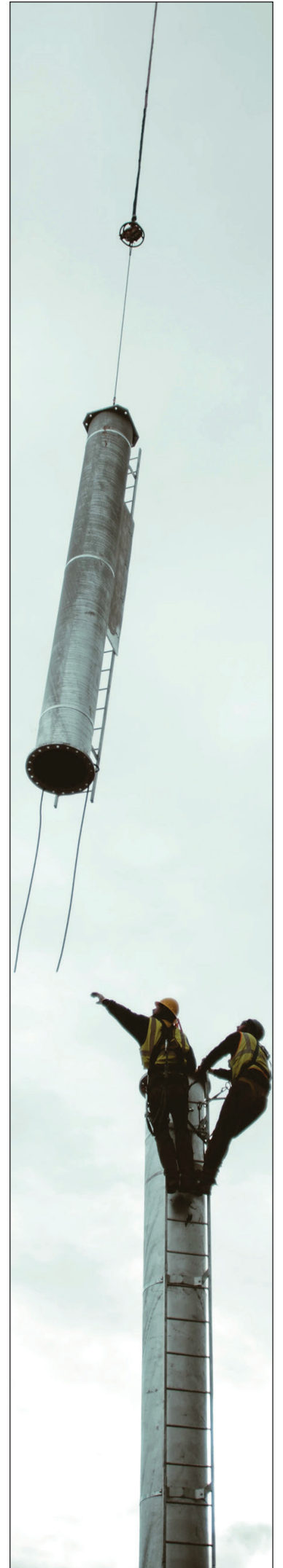
Workers for Utah-based lift manufacturer SkyTrac are currently installing new, fixed-grip quad chairlifts in Lefty's Canyon and Mary's Bowl at Powder Mountain ski resort. Completion is scheduled for mid-December.
