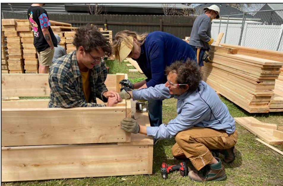
Volunteers construct planter boxes for one of Wasatch Community Gardens' neighborhood garden plots in Salt Lake City.
