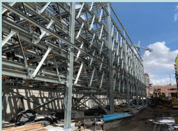
Paperbox Lofts APS Construction
