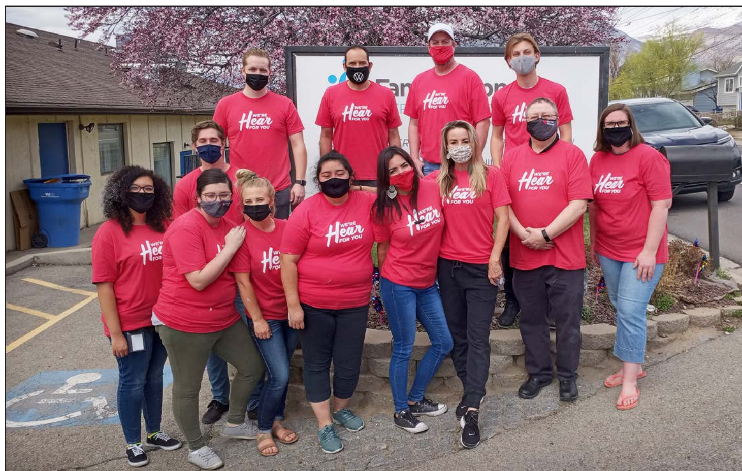
Through its We're Hear For You program, Ken Garff Automotive Group is renovating several play therapy rooms at the Family Support and Treatment Center. Ken Garff employees have been working hands-on doing demolition, painting and more. Photo courtesy of the Family Support and Treatment Center.
