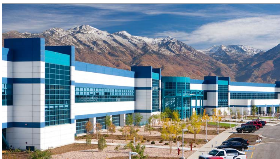
When Micron Technology decided to discontinue manufacture of its 3D XPoint memory chip, its 2 million-square-foot Lehi factory was idled. Texas Instruments has now bought the facility and will covert it to manufacture its own 300-millimeter wafer computer chips.
