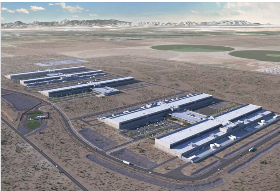
A rendering of the Facebook data center in Eagle Mountain, Utah. The facility is situated with the Sweetwater Industrial Park.
