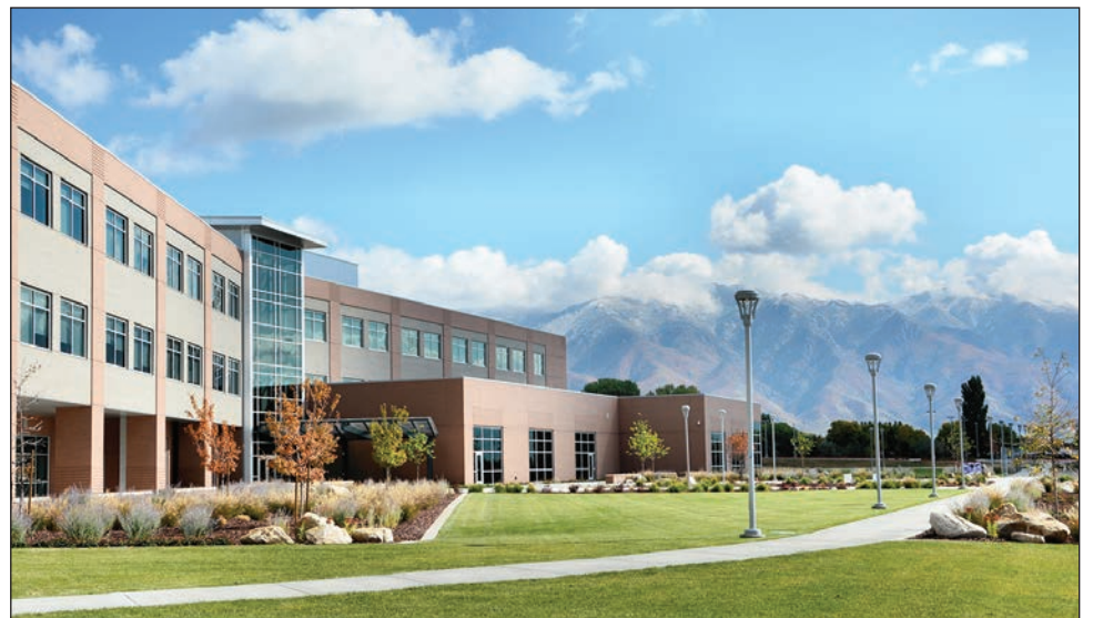
Weber State University, Davis Campus, is located in Layton. Weber State, Hill AFB and Layton celebrated the addition of a new Computer and Automotive Engineering Building in October 2020.
