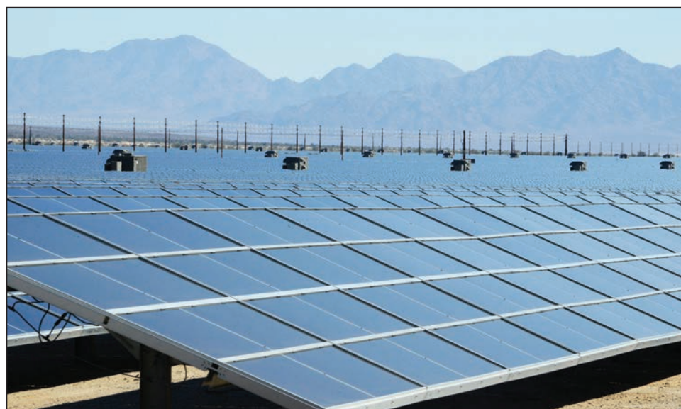
Rio Tinto has announced plans to build a tellurium extraction plant at its Bingham Canyon Kennecott copper mine. Tellurium is a component of cadmium telluride, a semiconductor used to manufacture thin film photovoltaic solar panels such as these at a solar power generating facility in Rich County.
