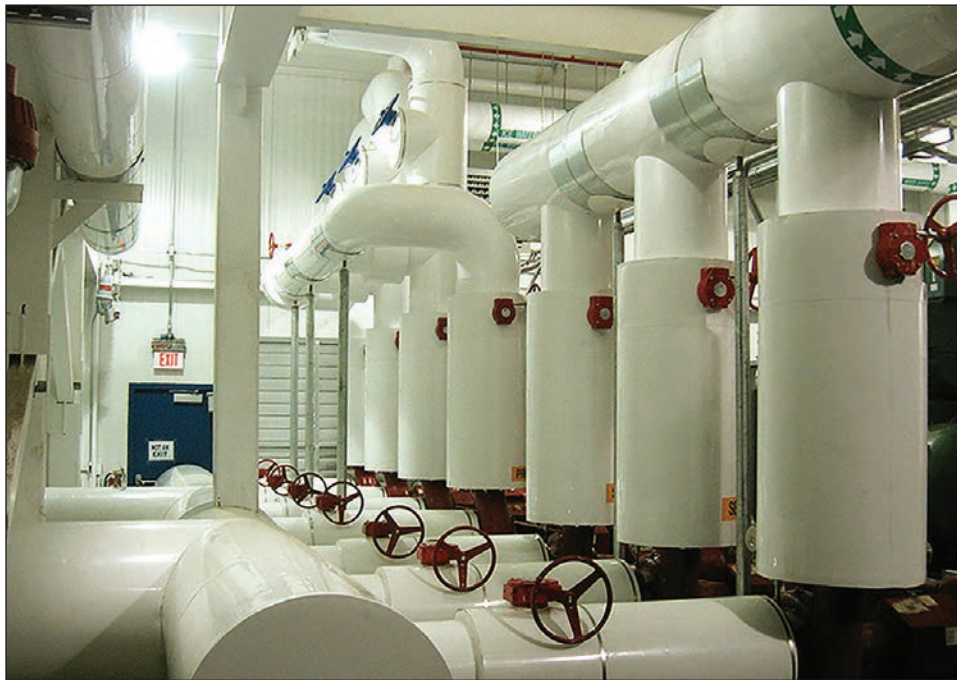
Raw materials are handled at the Dannon yogurt plant in West Jordan. A number of other food manufacturers are considering Utah as a site for operations, according to the Economic Development Corporation of Utah.
