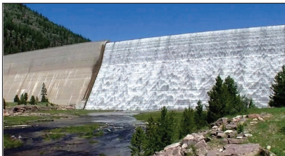
The spillway on the Upper Stillwater Dam in Duchesne County overflows following record-breaking precipitation in May 2015. The dam, part of the Bonneville Unit of the Central Utah Project, is one of dozens of major water-control installations around the state made by the project since its inception in 1960.
